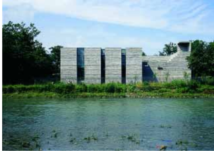
The facade of the Luyeyuan Stone Sculpture Art Museum, completed in 2002, consists of cast concrete. Its structure was created using slate slabs as formwork.
