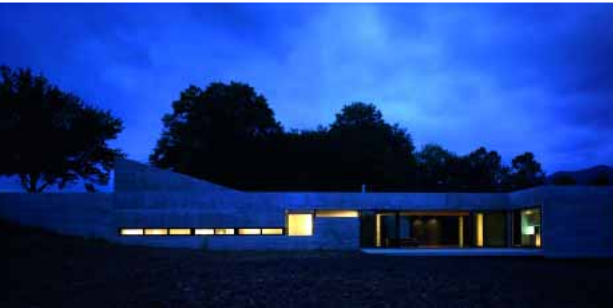
The town of Olot is located in the volcanic mountains of northern Catalonia. A little way outside of town, in Vall de Bianya, can be found "Casa Bianna", a long, one-storey private home. Strip windows emphasise the shape of the structure.
