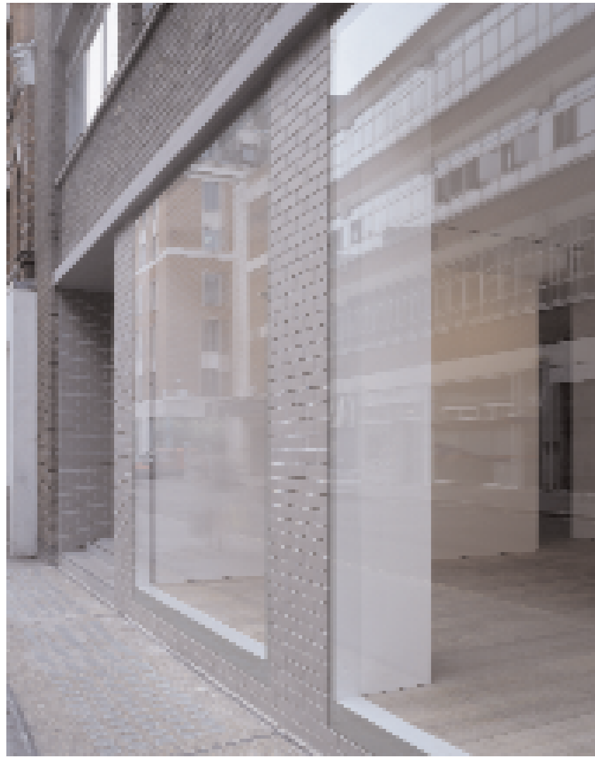
Above The facade, formerly recessed behind columns, has been brought forward to the building line. Plan/cross section The gallery occupies the ground and basement levels of the existing building; the 540sq m project cost £380,000 and was on site for 12 weeks.
