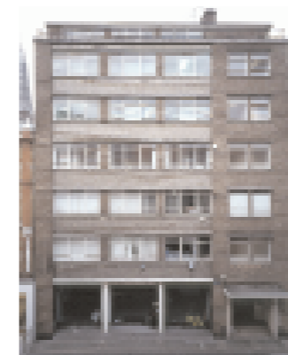
Above The gallery features full-height glazing to the Eastcastle Street frontage. Below/right 'Before'; axonometric.
