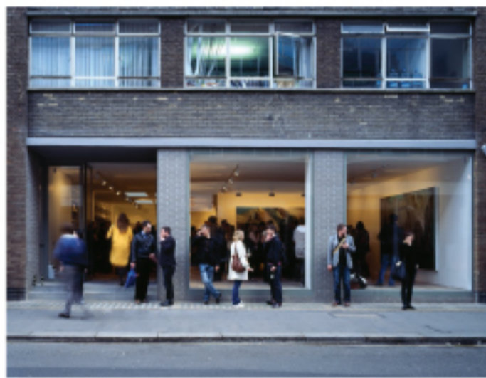
Brick piers align with those of the elevation above.
